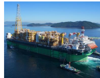
Egina FPSO (2013~2018, delivered)
